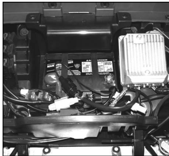
Fig. 12.1 (View with hood removed)
