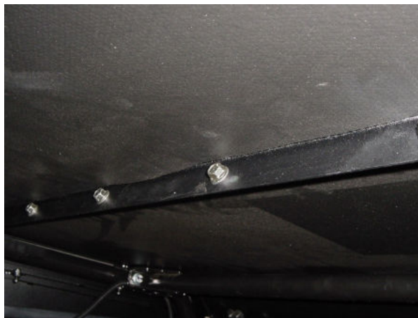
Fig. 8.4 (view of bolts between roof halves)
